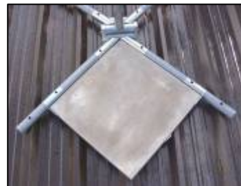
7. Check angles correct, tighten locking nuts
