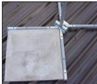
9. Fit paving slabs
