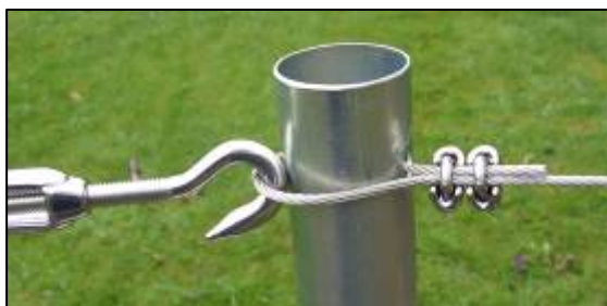
10. Fasten net support wire through holes at top of sleeve
